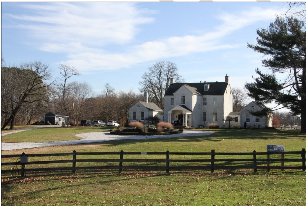
Figure 9: Sandy Point Farm House (AA-330), view southeast
