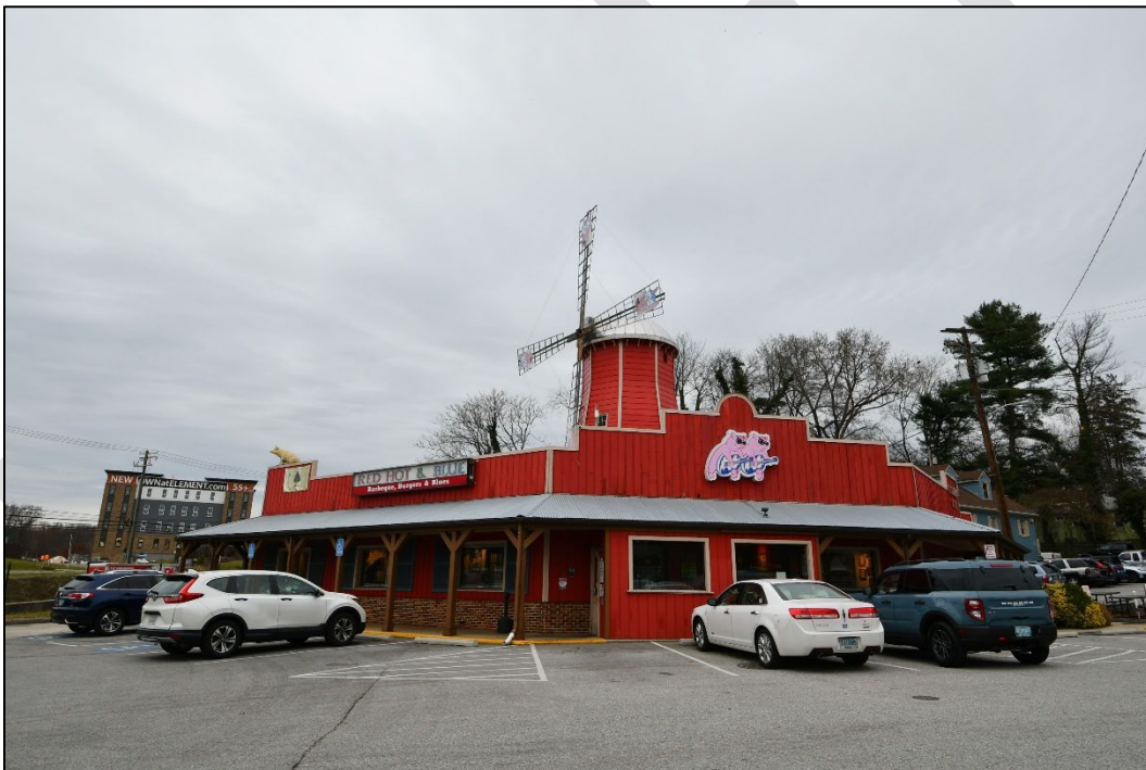
Figure 5: Dutch Mill Farm Restaurant (AA-2603), view north toward U.S. 50/301.
