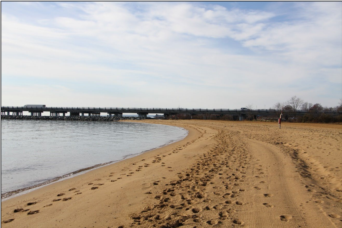
Figure 13: Sandy Point State Park (AA-2305), South Beach, and Chesapeake Bay Bridge, view southwest.
