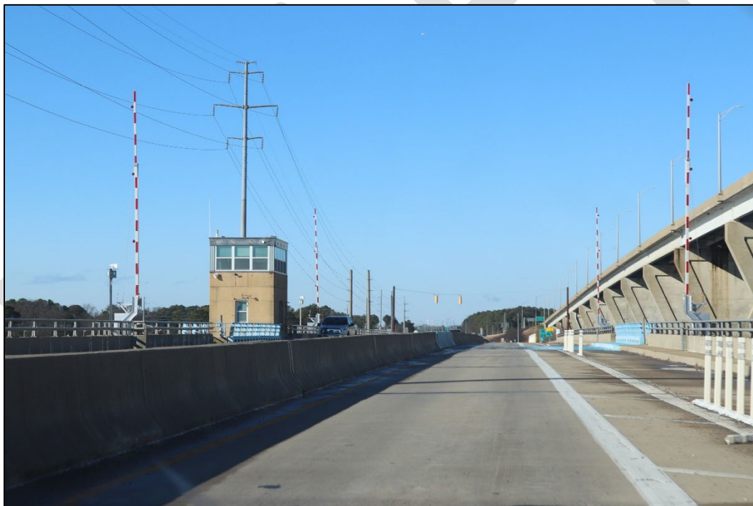
Figure 33: SHA Bridge 1700600 (QA-542), view west
