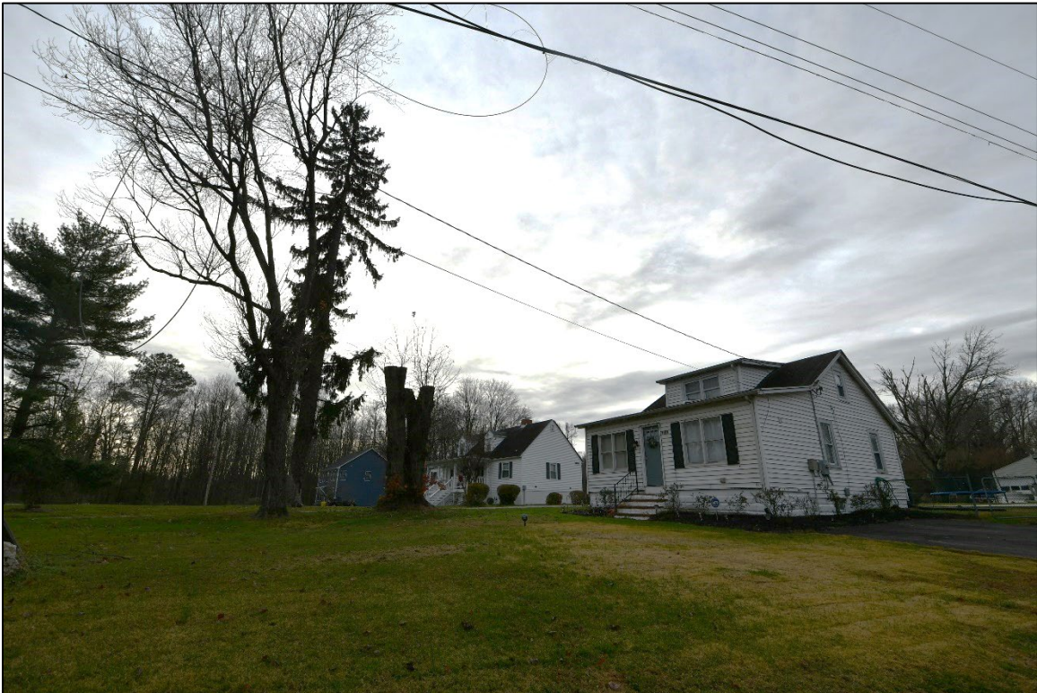
Figure 16: Skidmore, contributing resources at 1045 Skidmore Drive (left) and 1601 Col-Mar Lane, view southeast.
