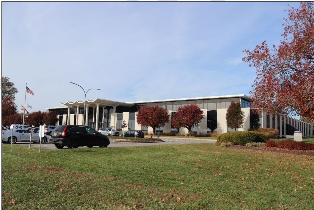
Figure 21: Westinghouse Ocean Research and Engineering Center (AA-2592), view west
