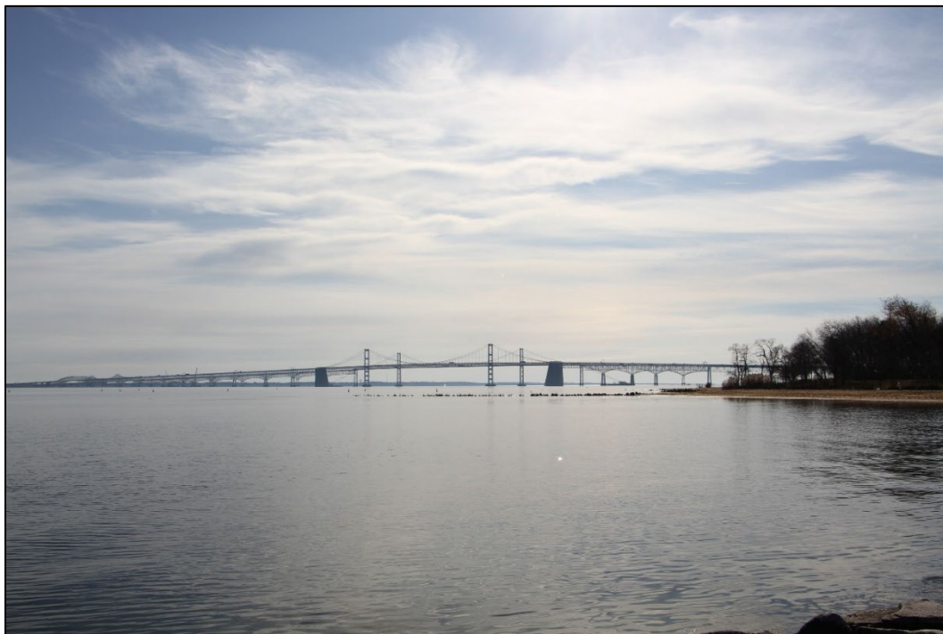
Figure 3: Chesapeake Bay Bridge (AA-47, AA-48), view southeast from Sandy Point State Park.
