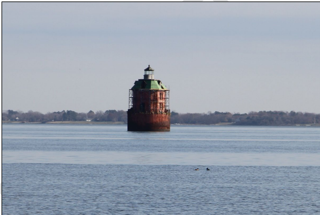
Figure 11: Sandy Point Light Station (AA-166), view from Sandy Point State Park
